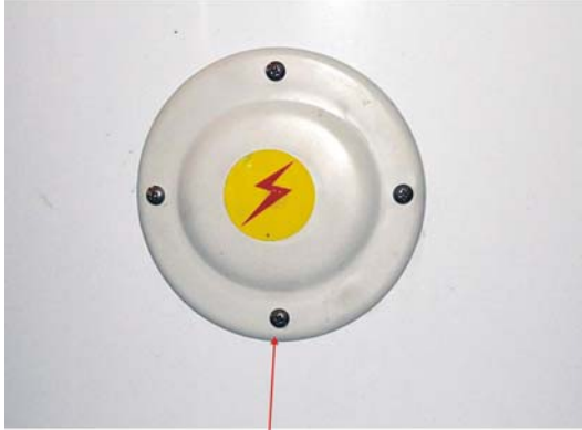
Remove the screw, and take away cover for electrical heater
